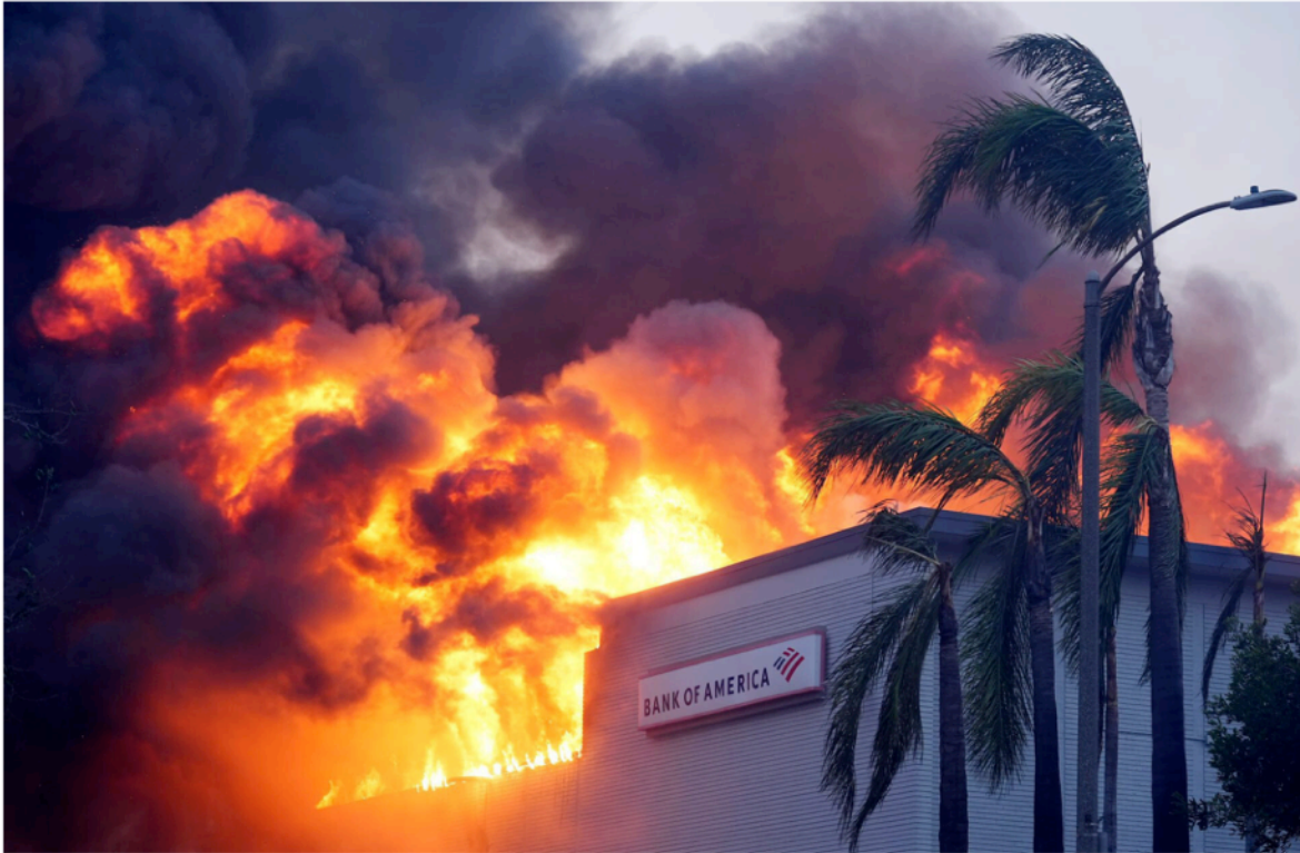
Flames engulf a Bank of America building in Altadena during the Eaton Fire on Jan. 8. (Chris Pizzello/AP)
